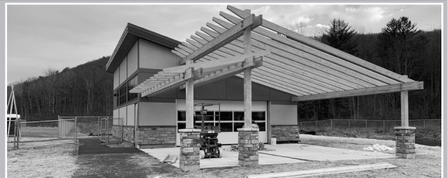
The Outdoor Learning Center is nearly complete.
